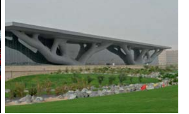
Qatar National Convention Center Doha / Qatar
